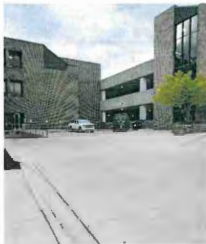
Photo 10: South Side Gannon Deck – looking northwest at structure and Gannon building
