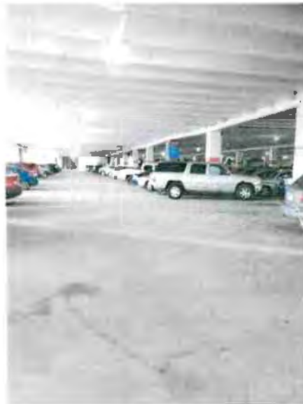
Photo 11: 1 st Level Gannon Deck – looking south
