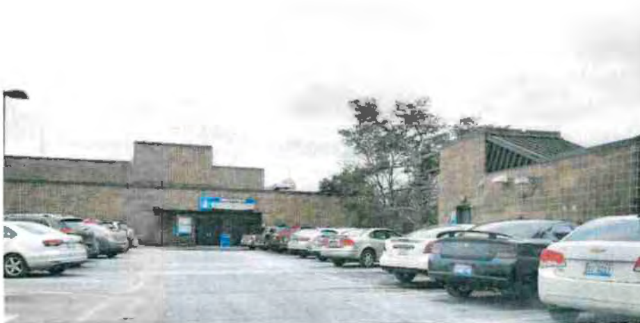
Photo 12: 3 rd Level Gannon Deck – looking south
