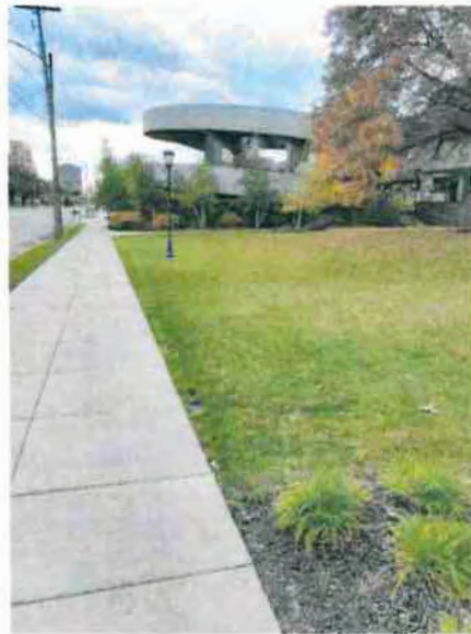
Photo 9: West Side Gannon Deck – looking south at helix exit ramp
