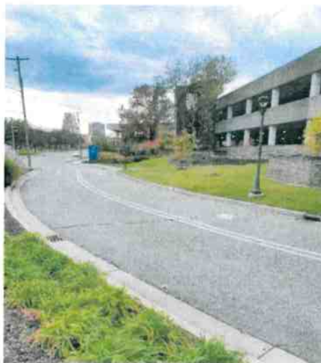
Photo 4: West Side Gannon Deck – looking south along Gannon Deck Entrance
