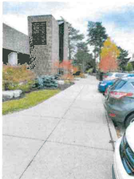
Photo 6: Eastern Project Limits – looking south along Gannon Deck
