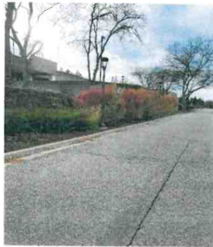
Photo 7: North Property Limits – looking west along Schoolcraft
