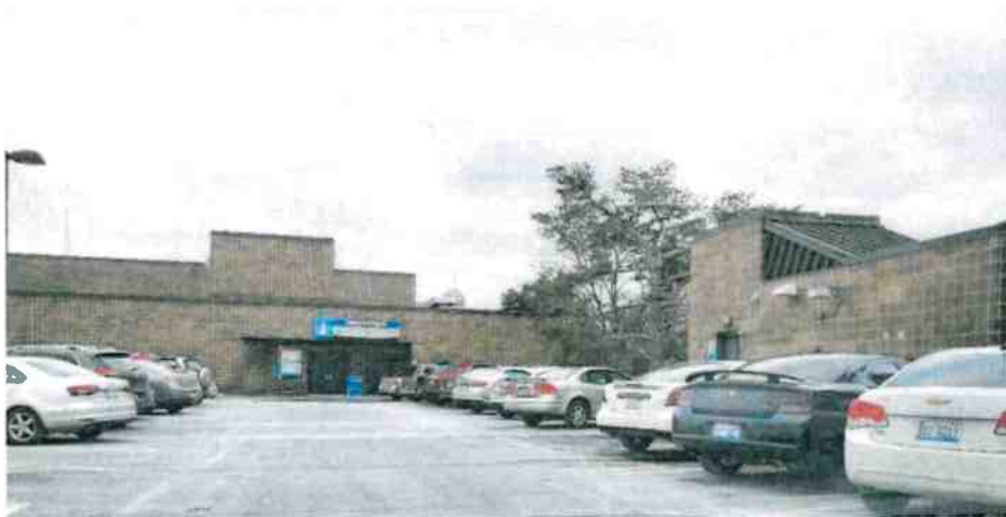
Photo 12: 3 rd Level Gannon Deck – looking south
