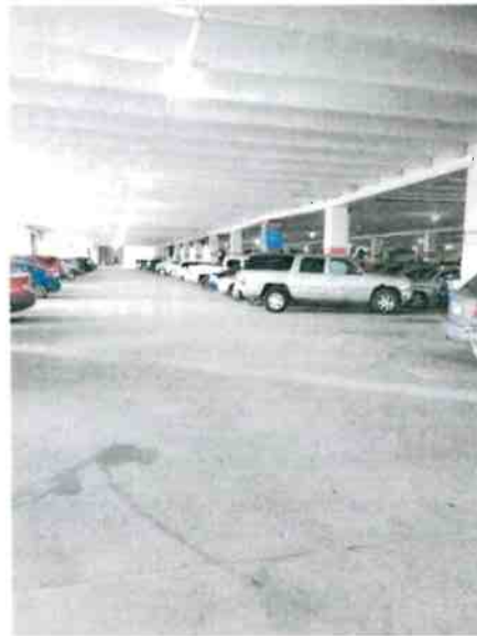
Photo 11: 1 st Level Gannon Deck – looking south
