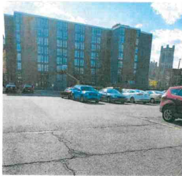
Photo 8: Southern Property Area – looking south at adjacent Oliver Towers
