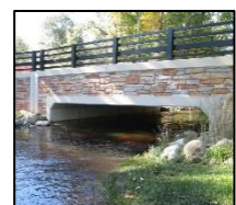
Figure 4: Three-sided box bridge
