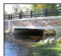
Figure 4: Three-sided box bridge
