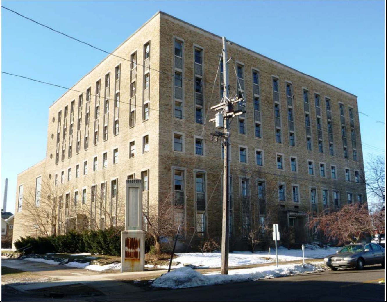
Existing YMCA Before Demolition
