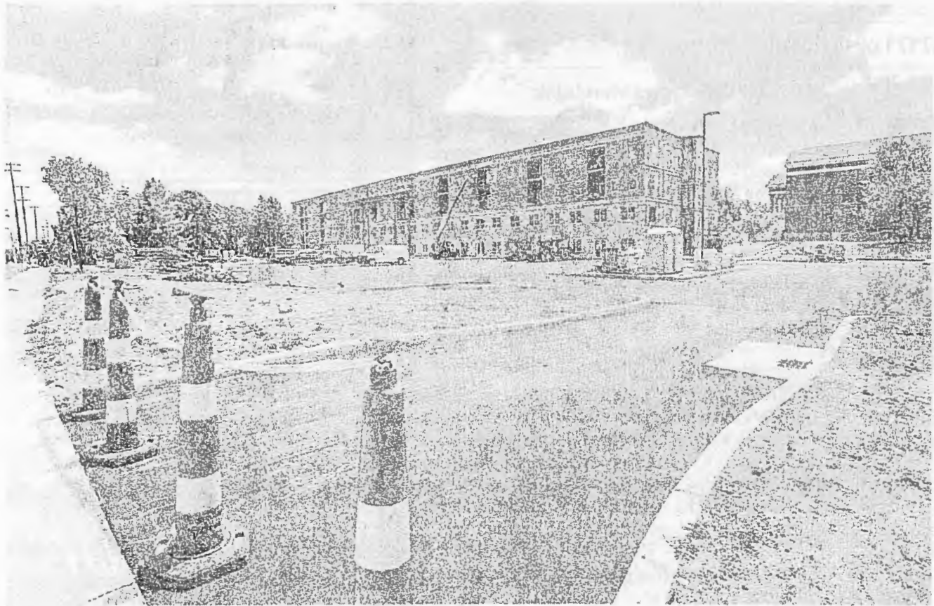
An Indianapolis-based developer has plans to redevelop the former Michigan School for the Blind site into three housing complexes. The 72-unit Walnut Park apartments project is currently under construction. MATTHEW DAE SMITH/LSJ
