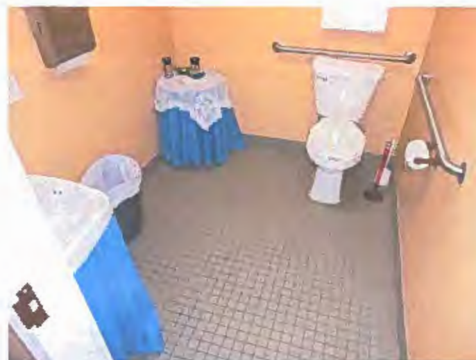
The leasing office restroom.
