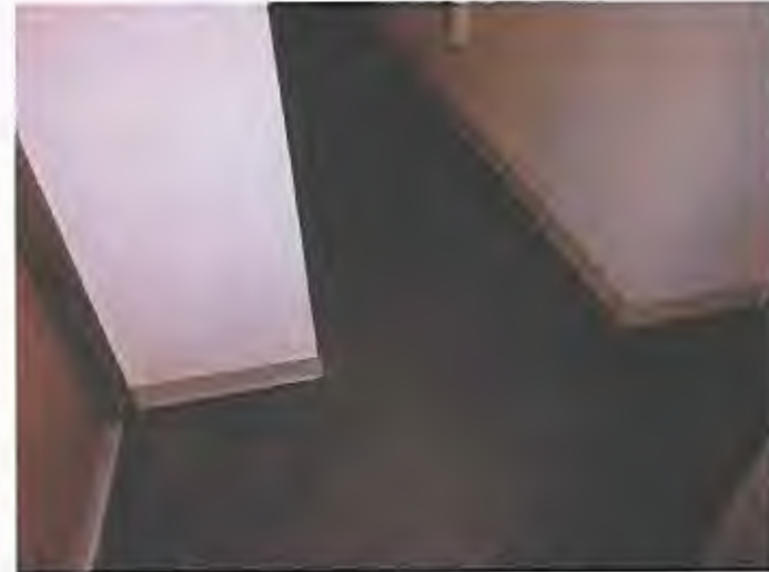
Typical common area hallway.
