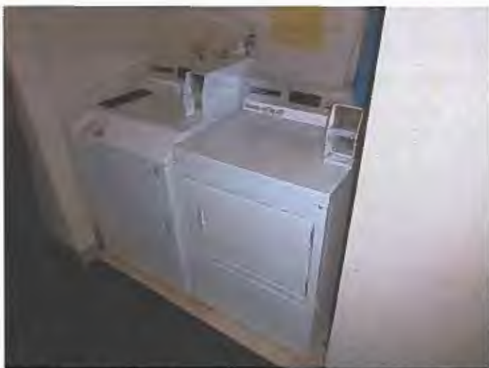
Each address feature a wash and dryer on the first floor level.
