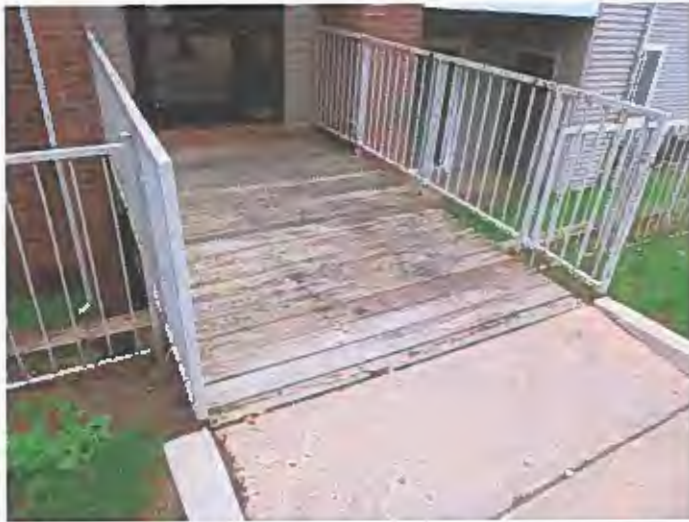
View of a pedestrian bridge providing access to the first floor.
