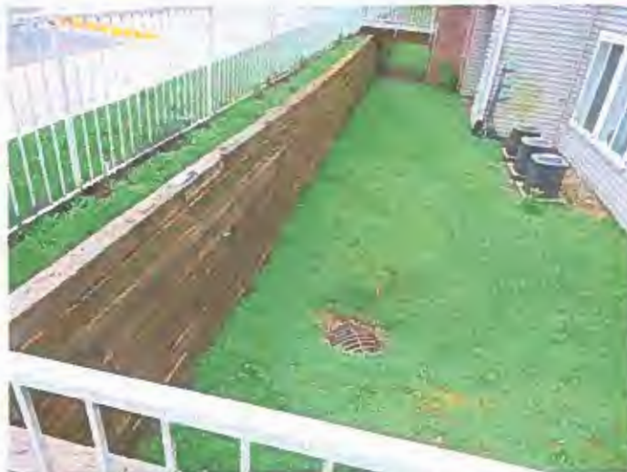
View of the wood retaining wall and steel railing system located at the front entrance of #623, #627 and #631.
