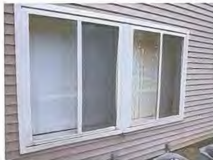
Typical aluminum-framed, slider type, double-pane windows.
