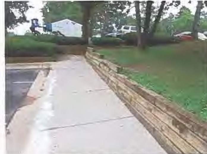
Typical concrete walkway conditions and example of timber retaining walls found throughout the site.
