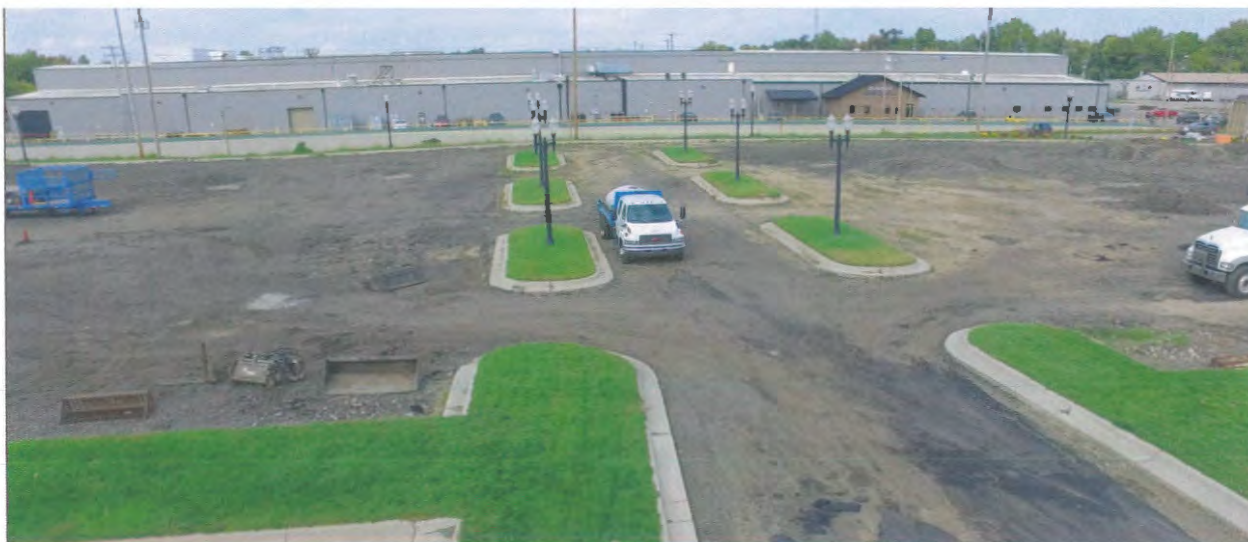
View from center of site looking North. Demmer is across Oakland viaduct.
