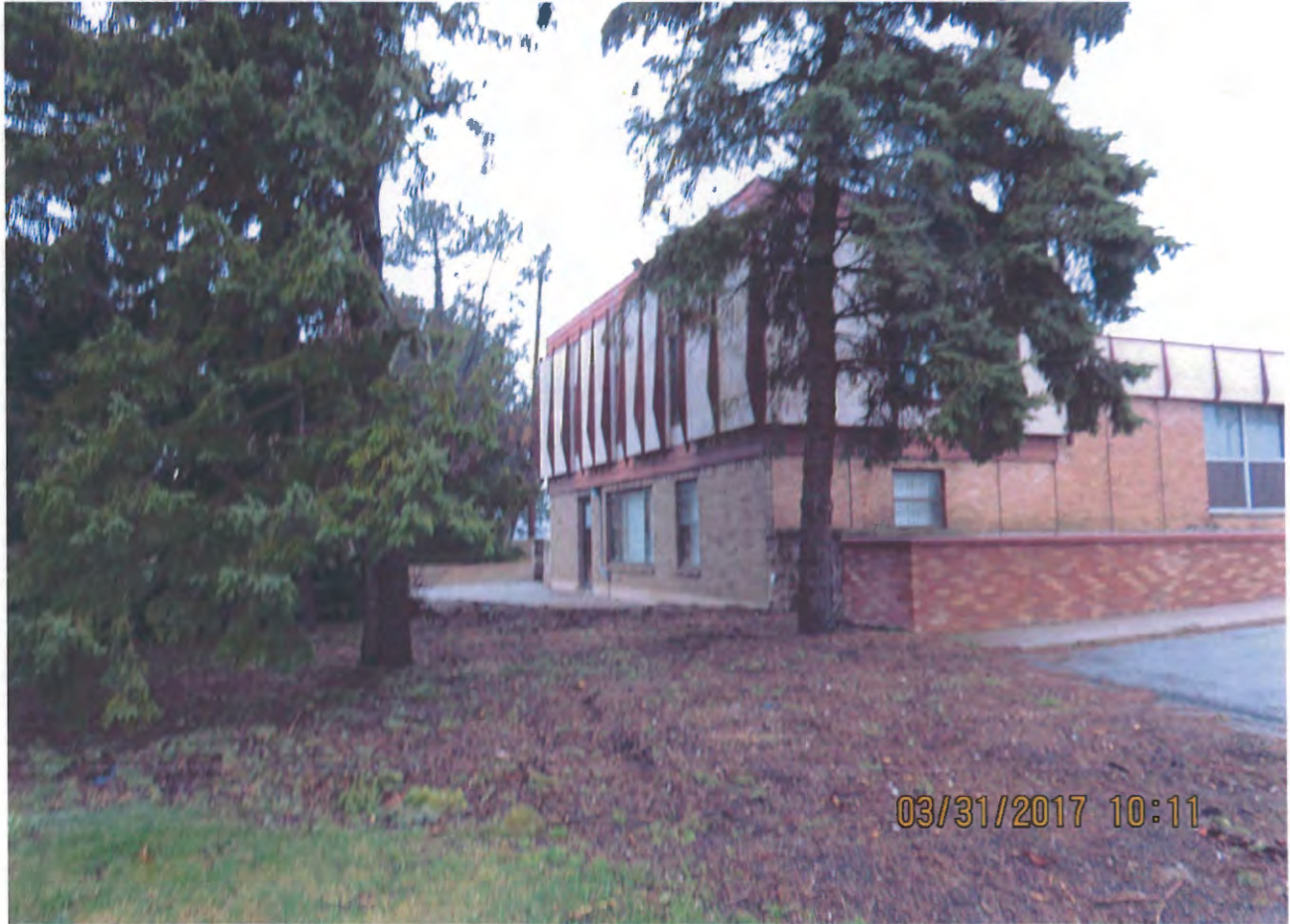
South East Corner
