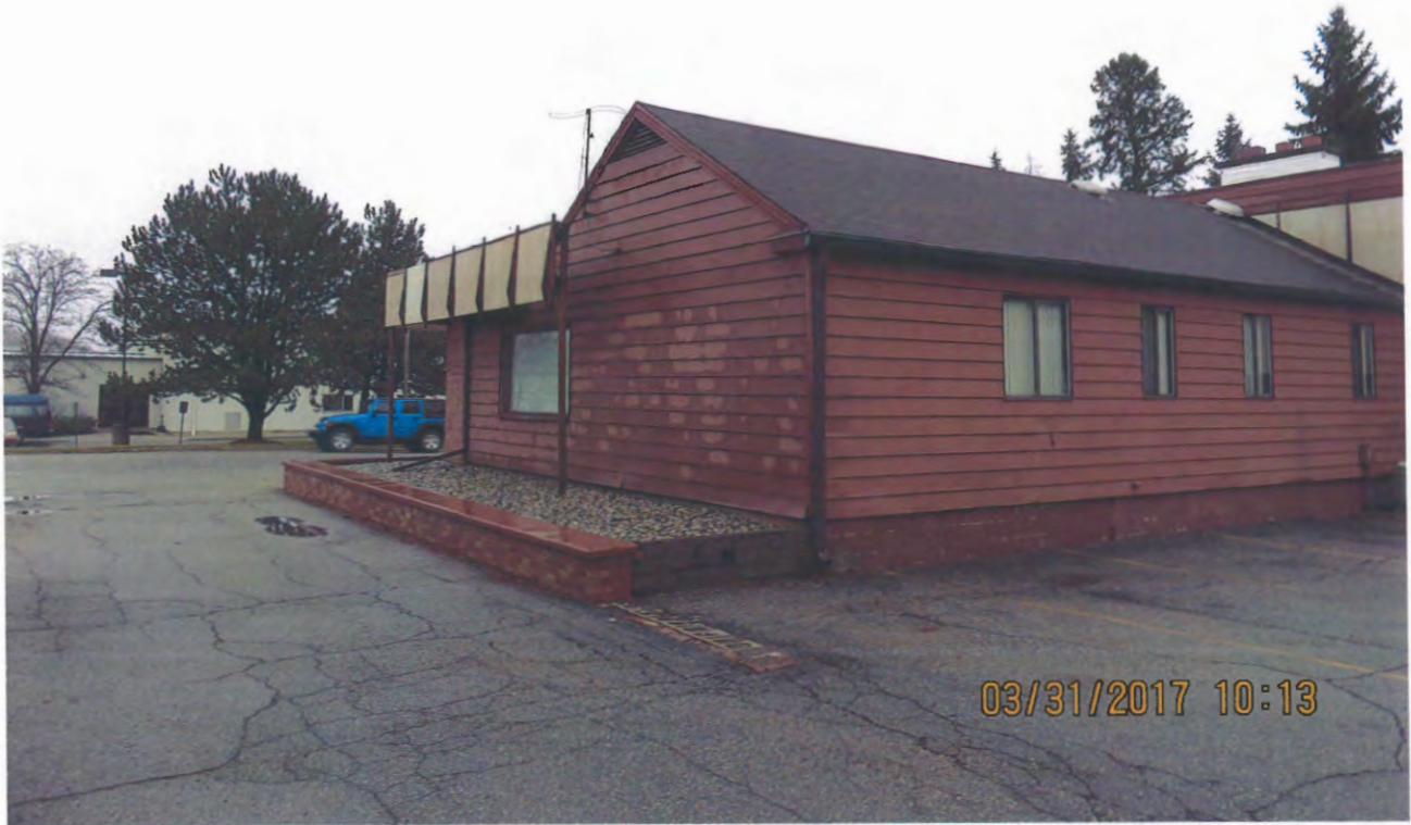
North West Corner
