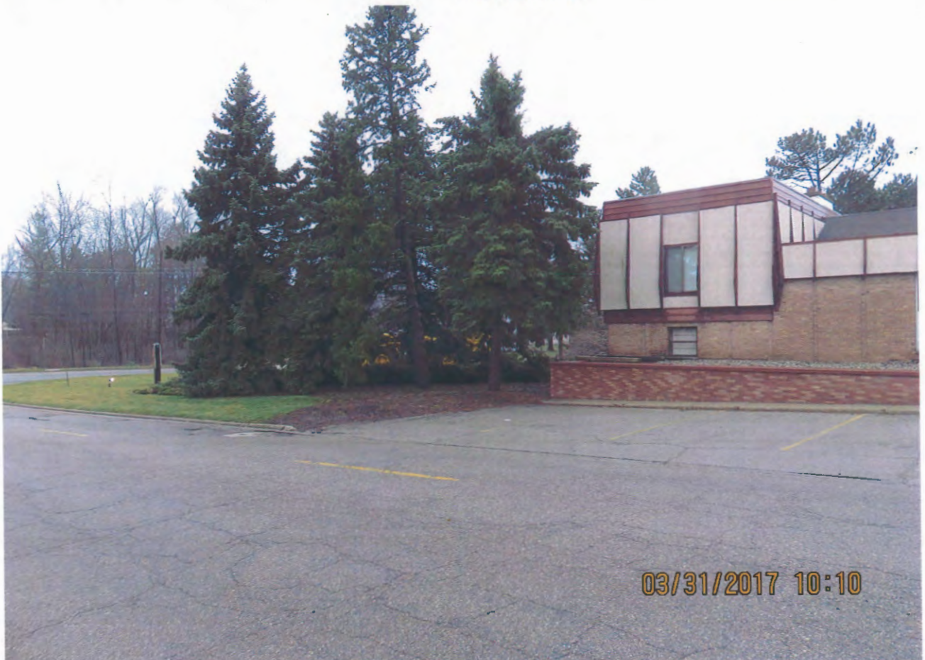
North Elevation (South end)
