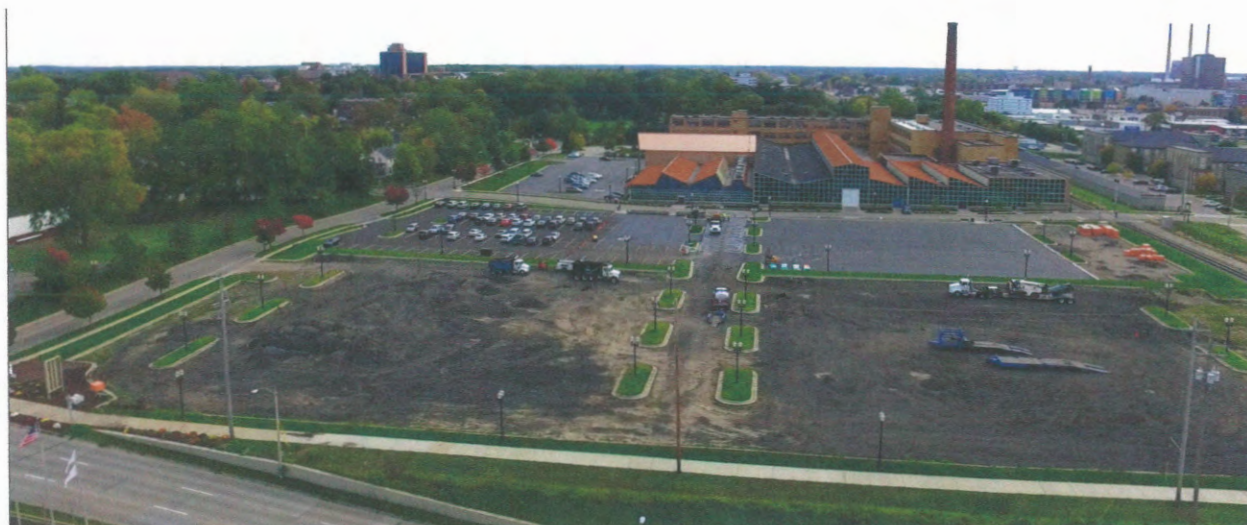
View from above Demmer looking South toward site.
