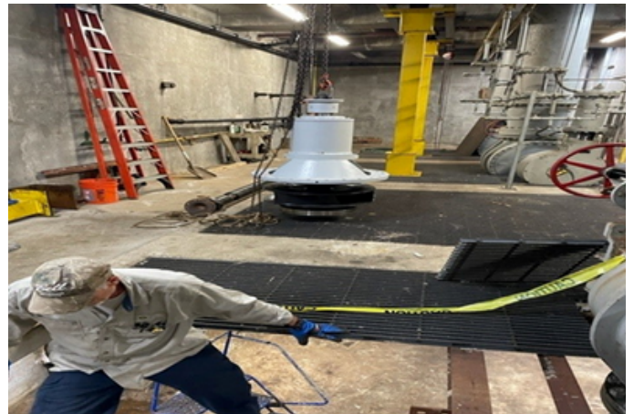
Maintenance Staff replacing South grit drive:
