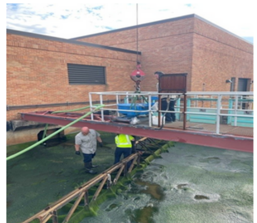
Maintenance Staff replacing South grit drive:
