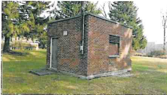
View of on Site municipal well pump house facing northeast.
