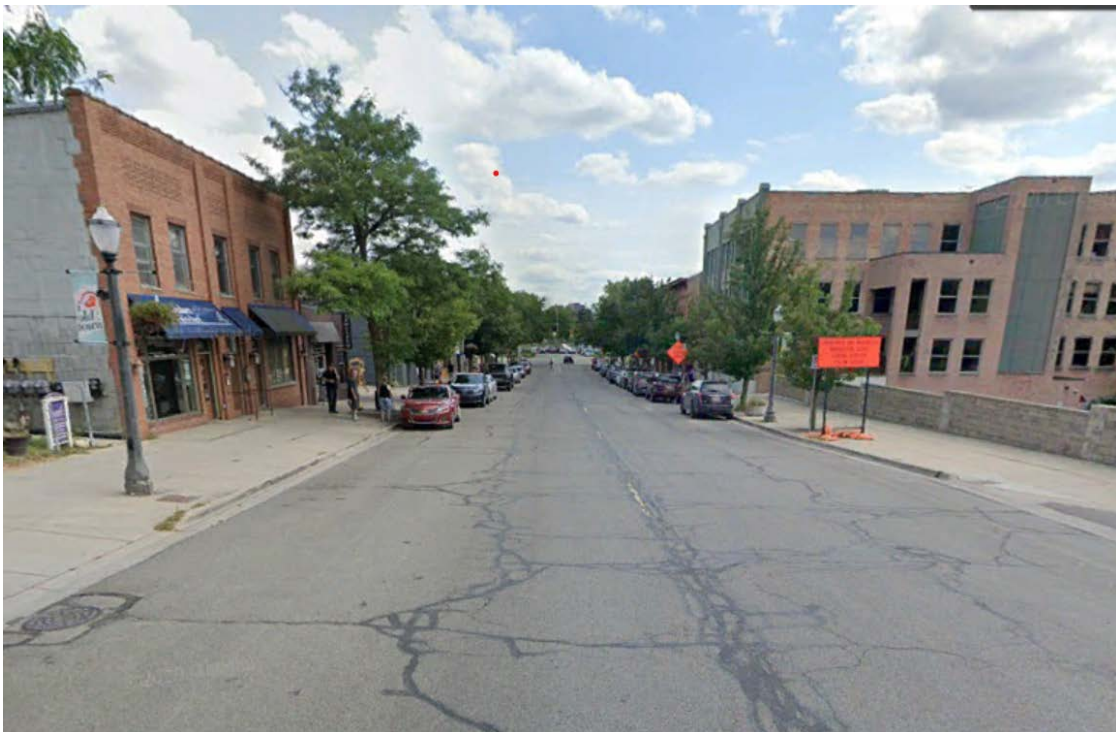
Turner Street at Clinton St. (Looking South towards Cesar E. Chavez Ave.)
