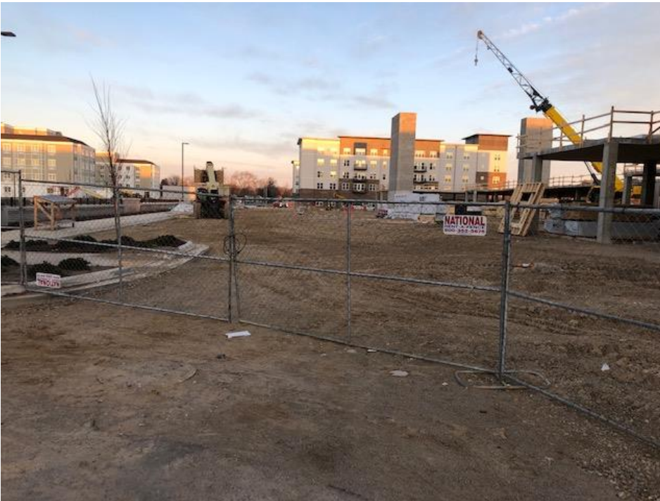
Josephine Lane under construction. Looking west from Cascade Boulevard. 3-29-2022
