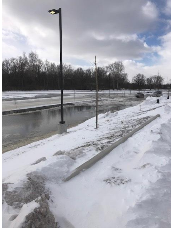
Red Cedar Parkway flooding 2-21-2022.
