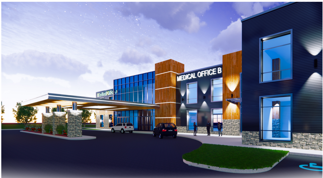
Building 1 - Elevation View Looking Southeast
