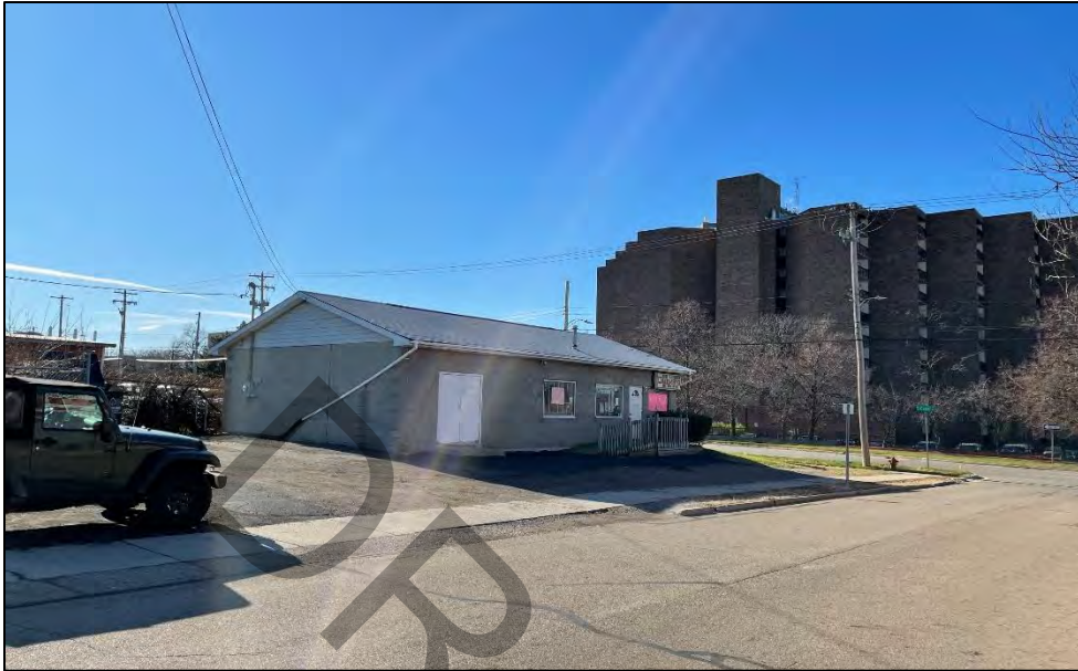
Photo 11: View of the north-adjointing site (Home Electronics – 538 N. Cedar Street, from Erie street, facing southwest.
