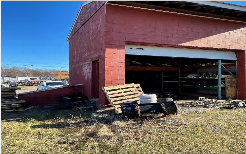
Photo 9: View of the garage building located in the northwest portion of the Property.
