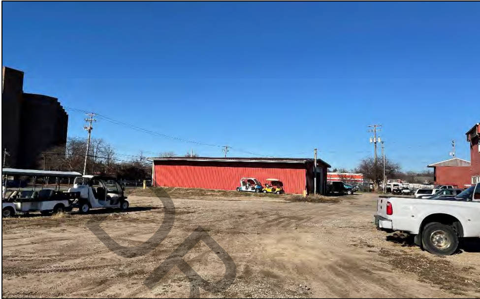
Photo 13: View of the south-adjointing site (southern portion of 500 N. Cedar Street) from the southern portion of the site, facing north.
