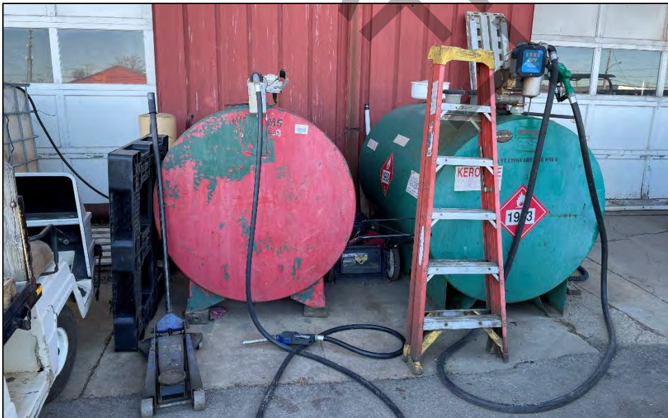
Photo 4: View of two above ground storage tanks located on the north side of the main service garage building.
