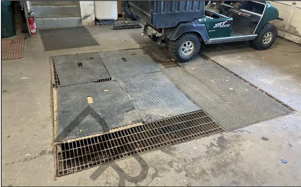
Photo 5: View of the trench drain located within the main service garage.
