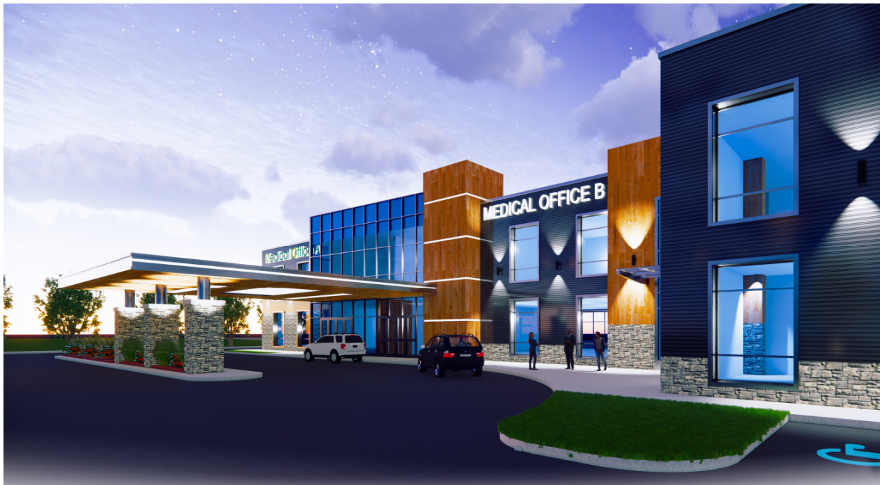
Building 1 - Elevation View Looking Southeast
