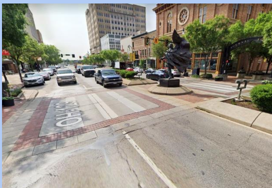
Figure 2-3 – Brick paved primary crosswalks as seen in Hamilton, OH. For more information, visit Case Studies on page 34.
