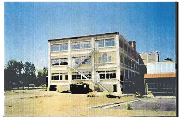
Prudden Wheel Condominiums
