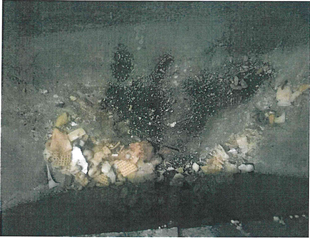
One of the registers I had to clean
