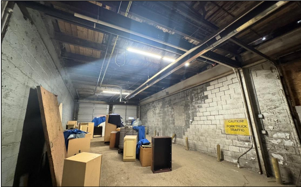
Photo 7: View within the subject property building.
