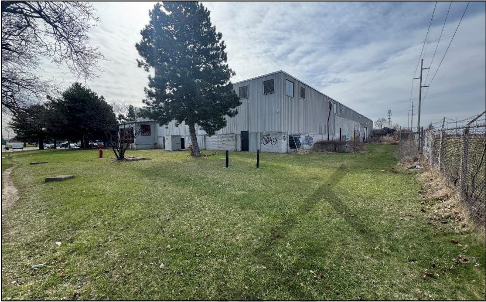
Photo 5: View to the southeast from the northeast corner of the subject property.
