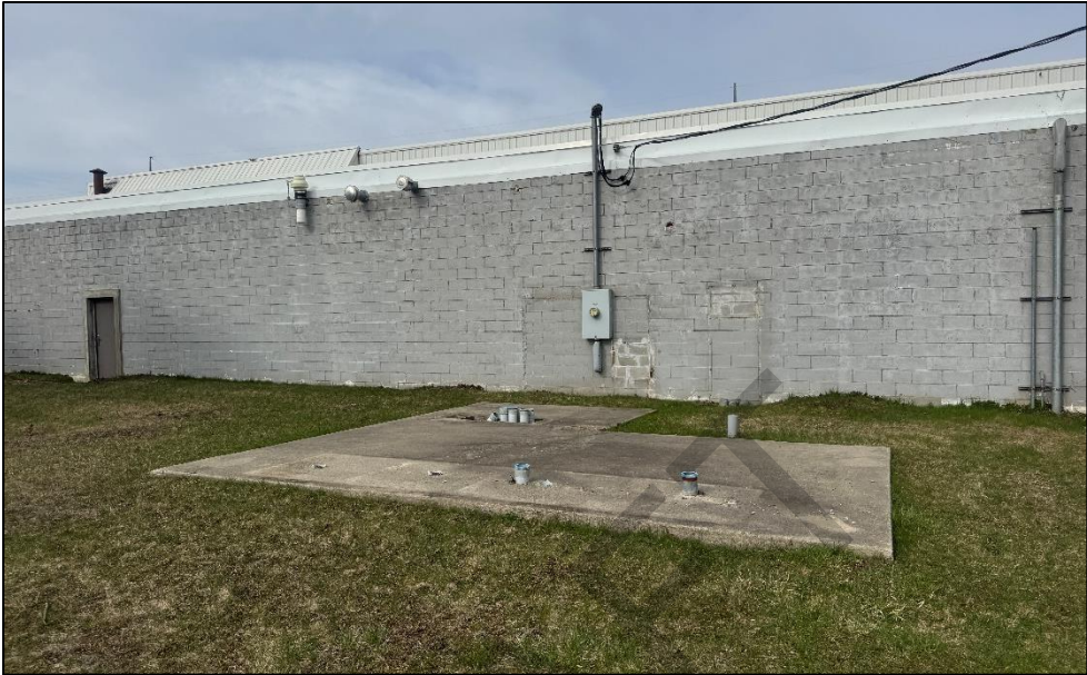
Photo 3: View to the west from the east side of the subject property.
