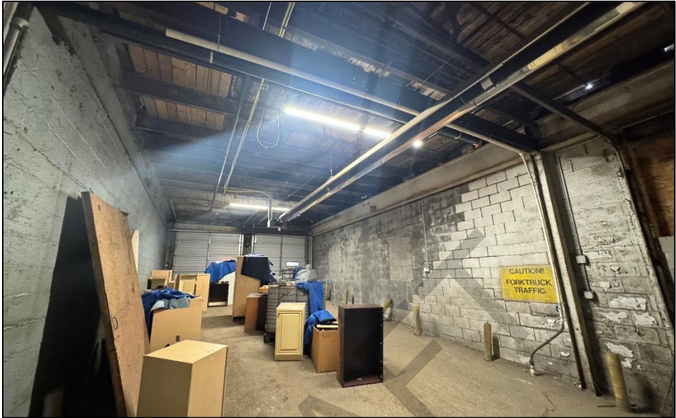
Photo 7: View within the subject property building.
