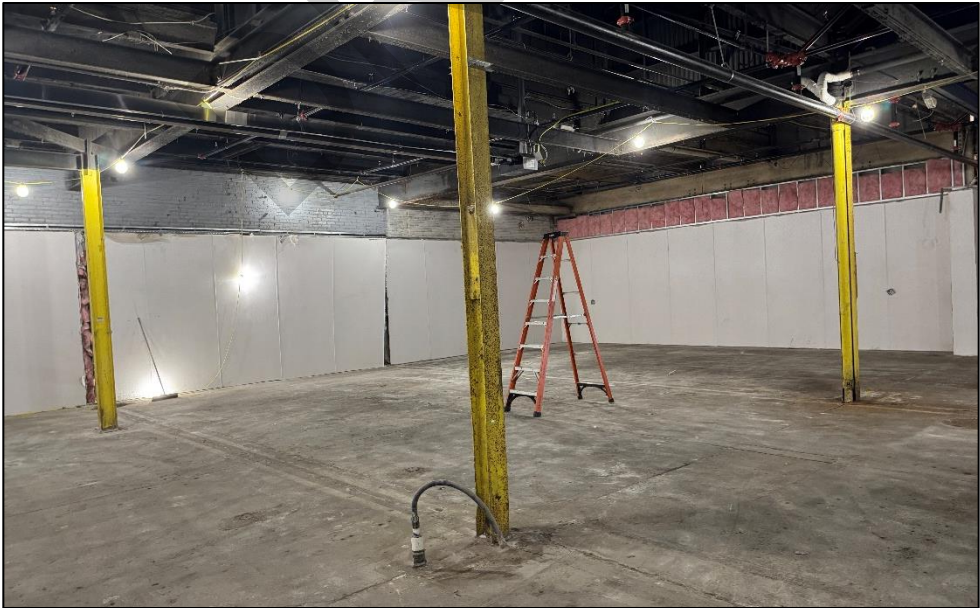
Photo 6: View within the subject property building.
