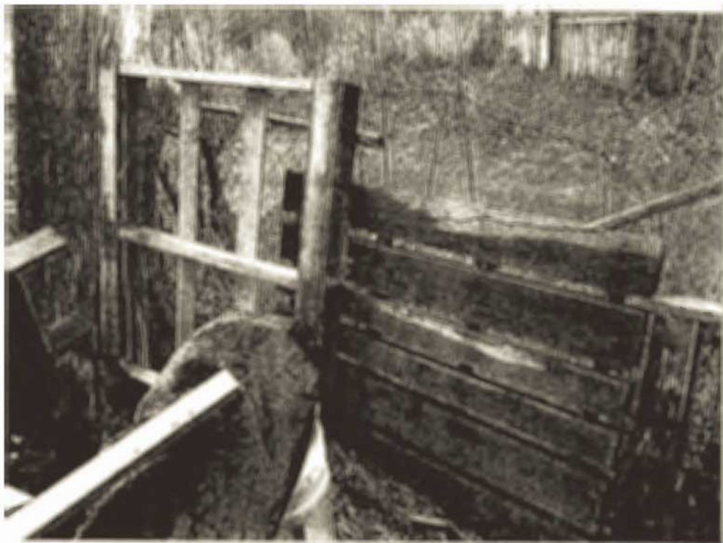
Covering hole in fence
