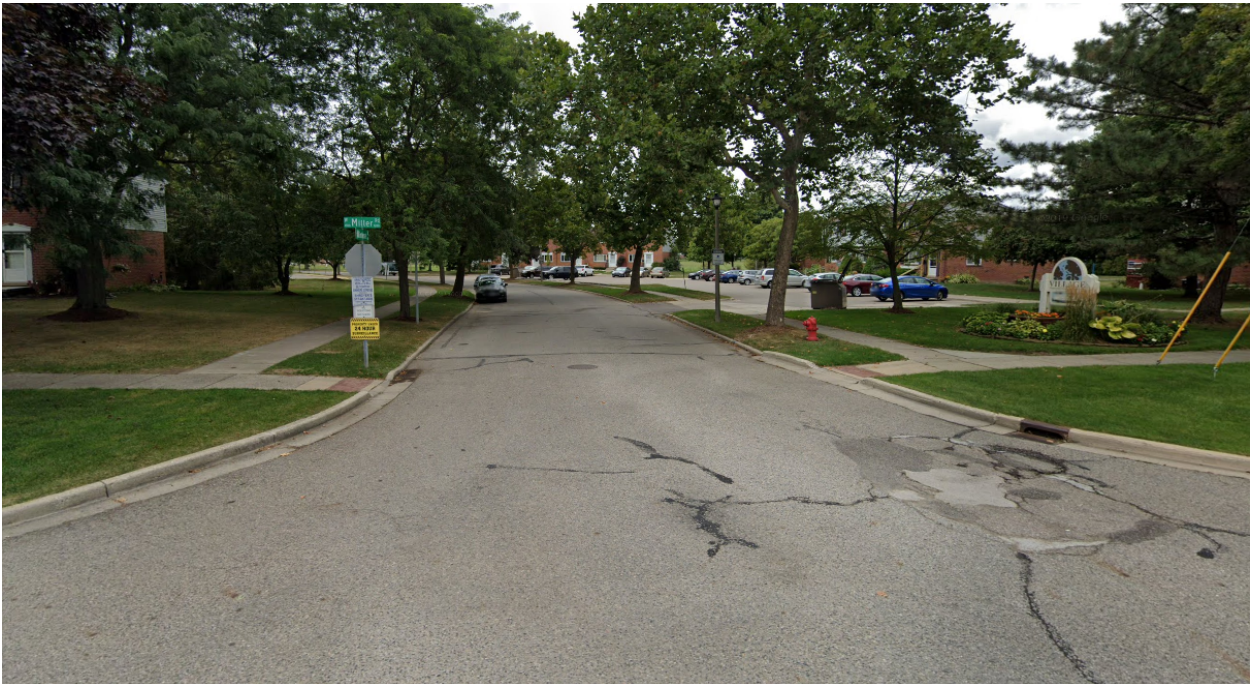
Winterset Drive – street view
