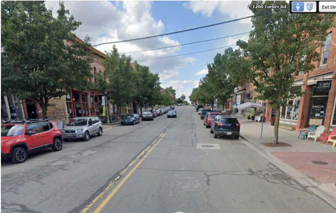
Turner Street at Cesar E. Chavez Ave. (looking north towards Clinton St.)
