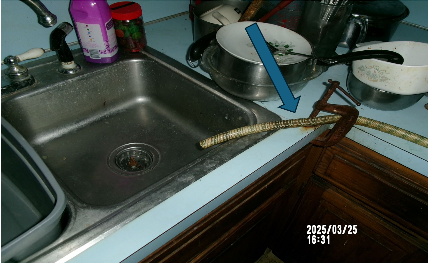
Hose clamped on counter with C clamp
