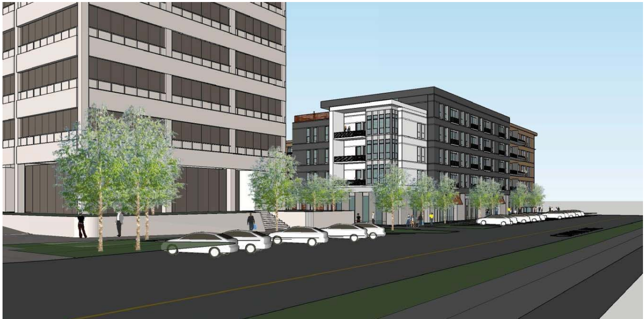
View Looking South along Capitol Avenue
