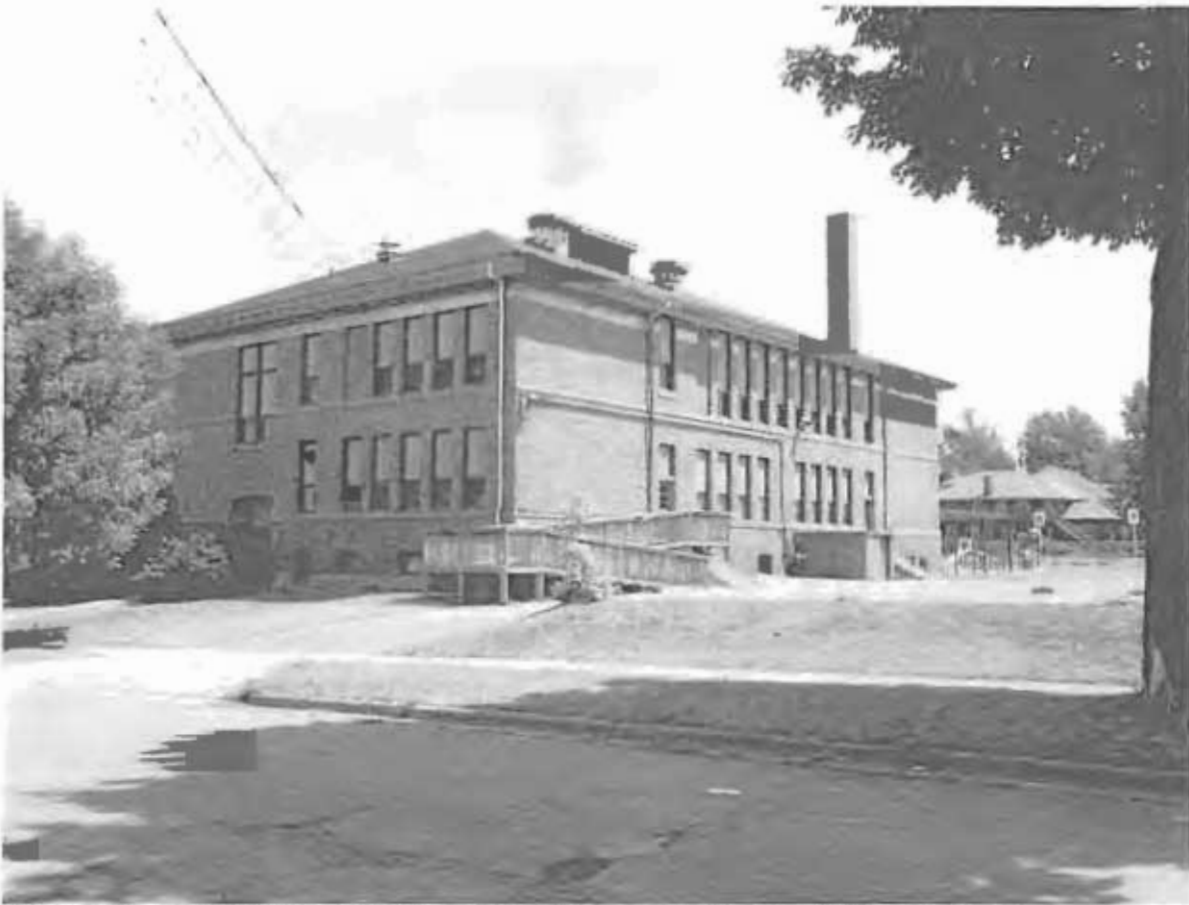
The Genesee Street Elementary School in 2013. Photo courtesy of MC Rothorn and the Downtown Neighborhood Association.
