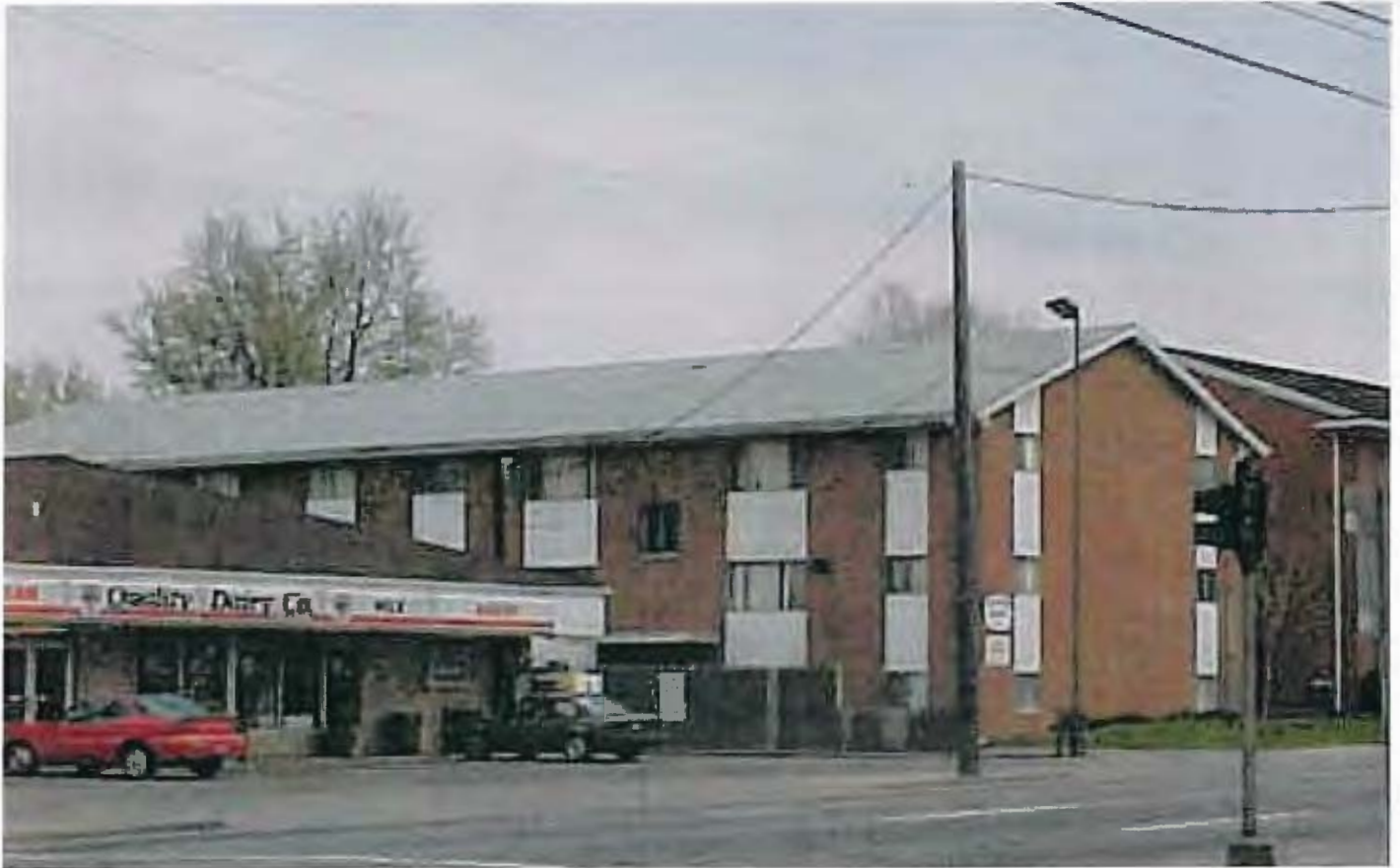
Apartment building at 516 W. Saginaw adjoining 714 N. Pine Street
