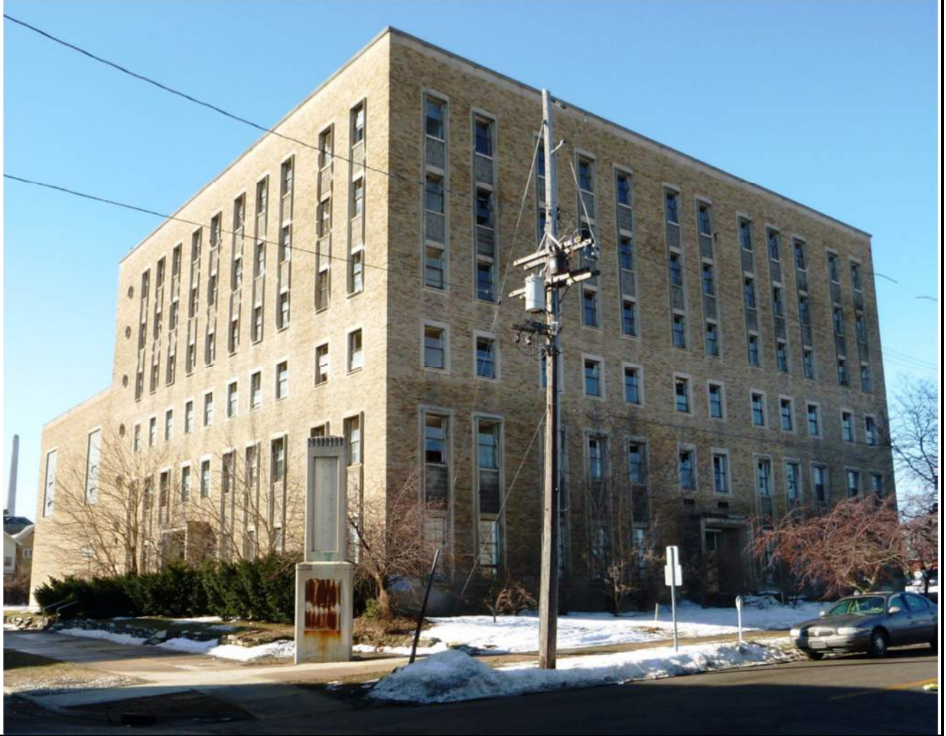
Existing YMCA Before Demolition
