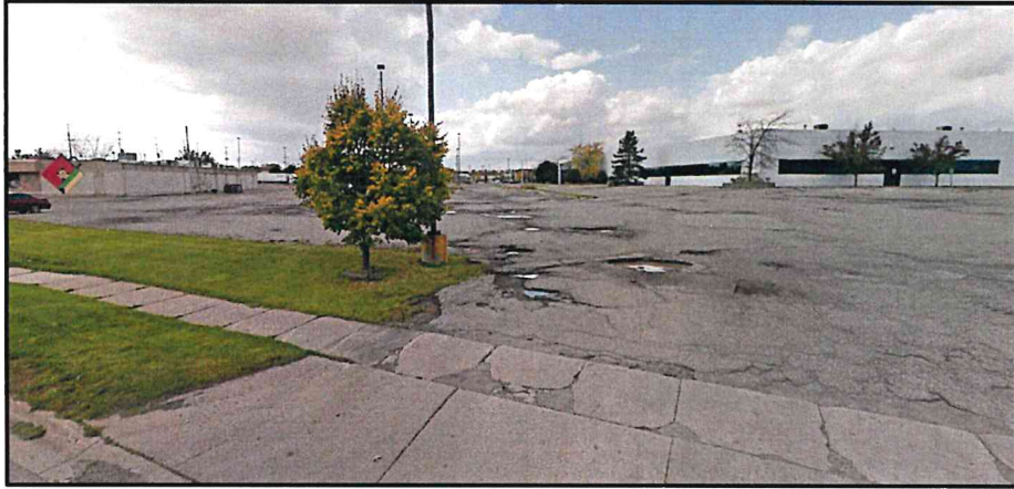
WASHINGTON ST LOOKING AT STORAGE LOT
