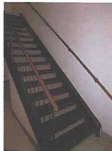
View of a common stairwell, railing system and rubber stair treads.
