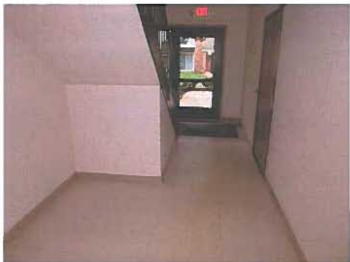
View of a typical common hallway/stairwell entrance.
