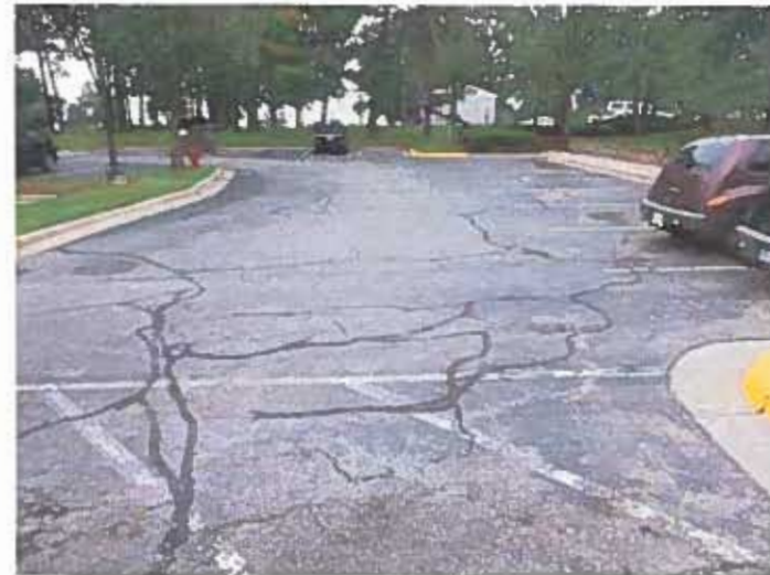
Typical condition of the asphalt paved parking lot areas.
