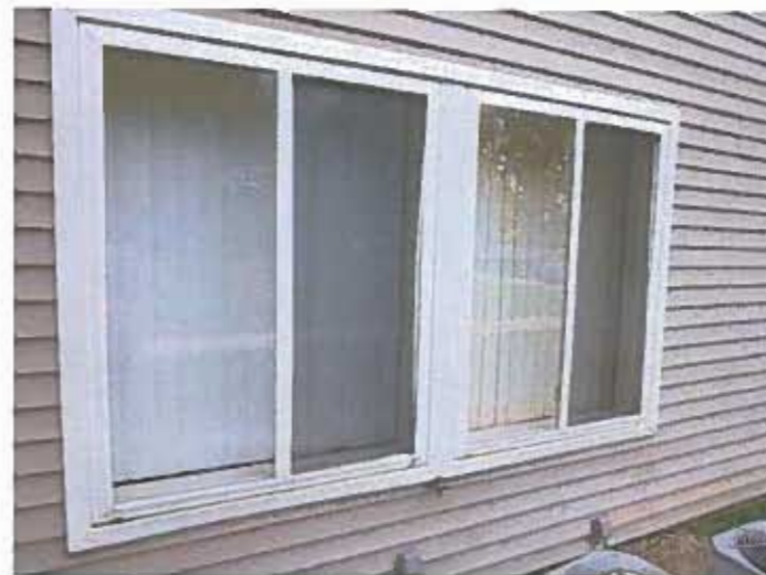
Typical aluminum-framed, slider type, double-pane windows.
