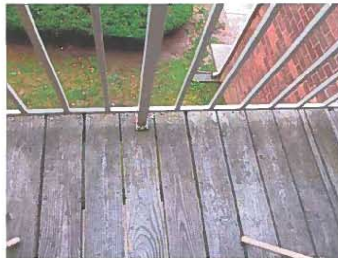
Close up of balcony decking.
