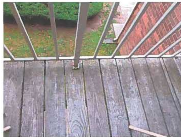
Close up of balcony decking.
