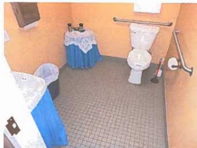
The leasing office restroom.
