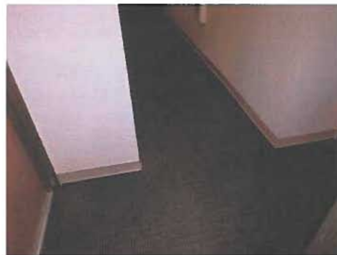
Typical common area hallway.
