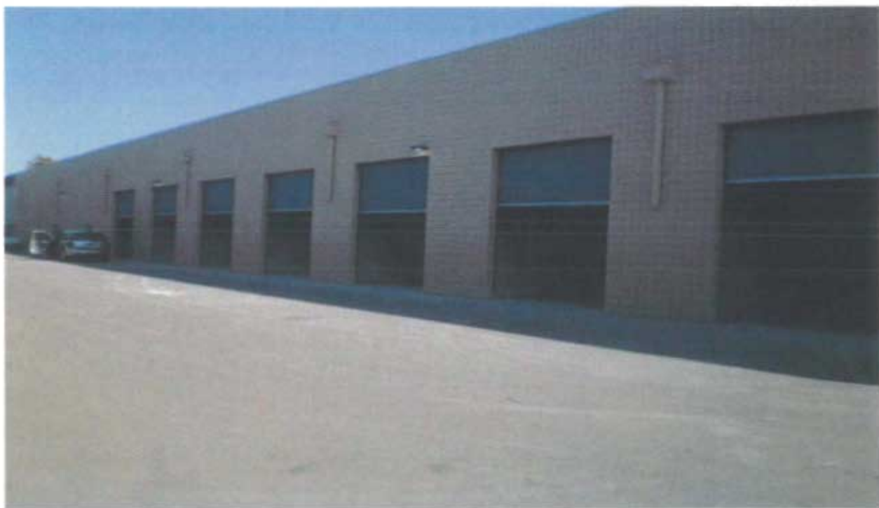
Rear Storage Units
