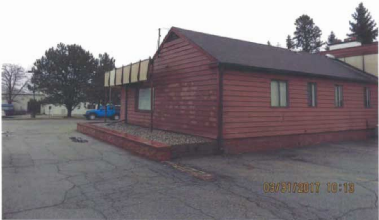
North West Corner
