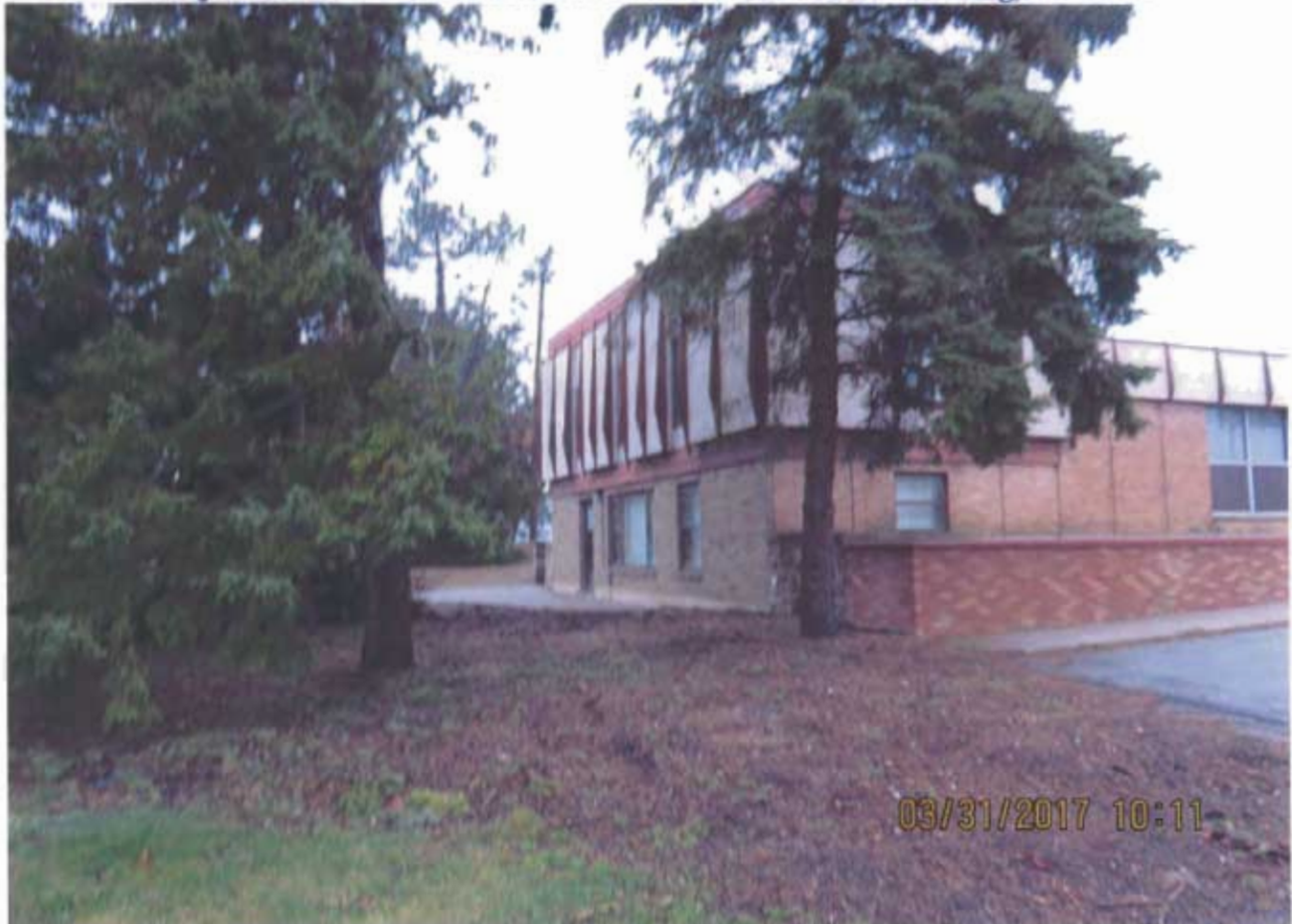
South East Corner
