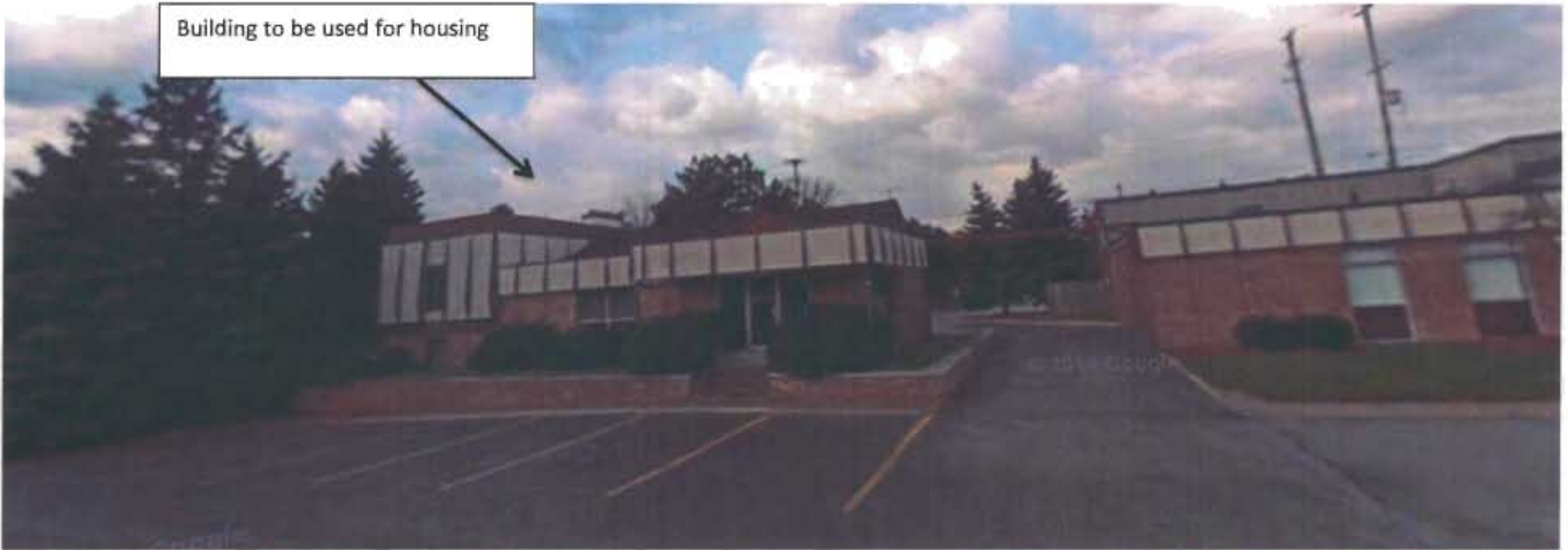
Vocational School Building
