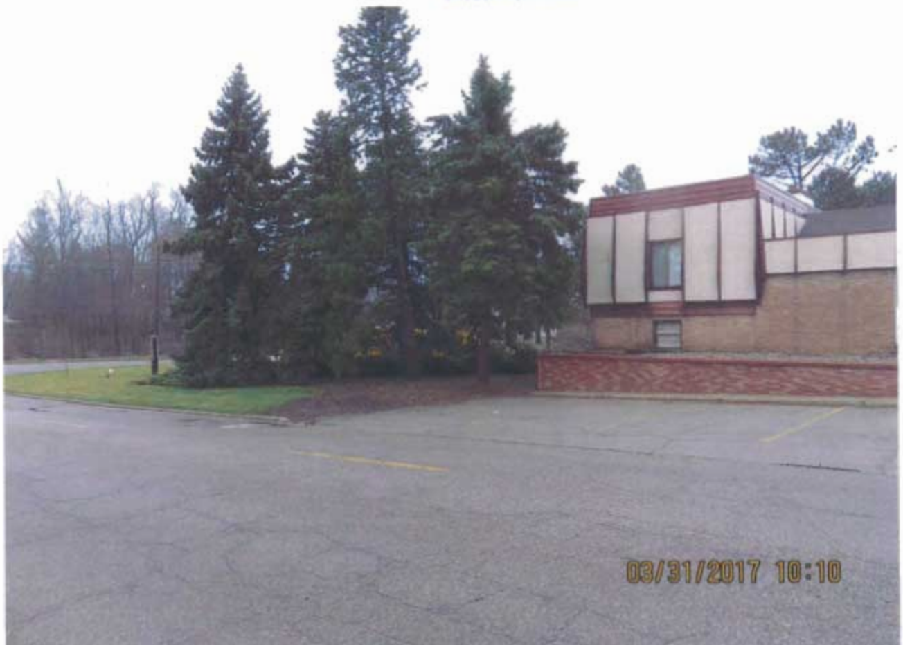
North Elevation (South end)
