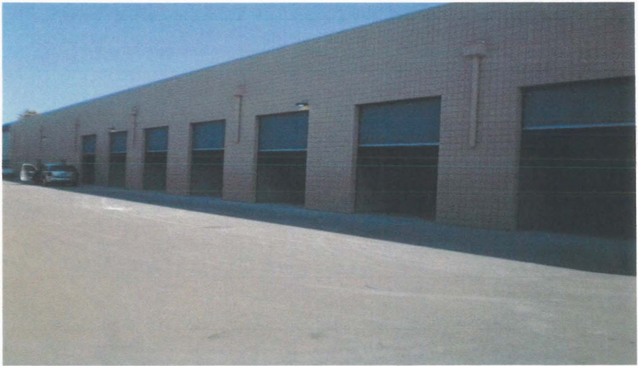
Rear Storage Units
