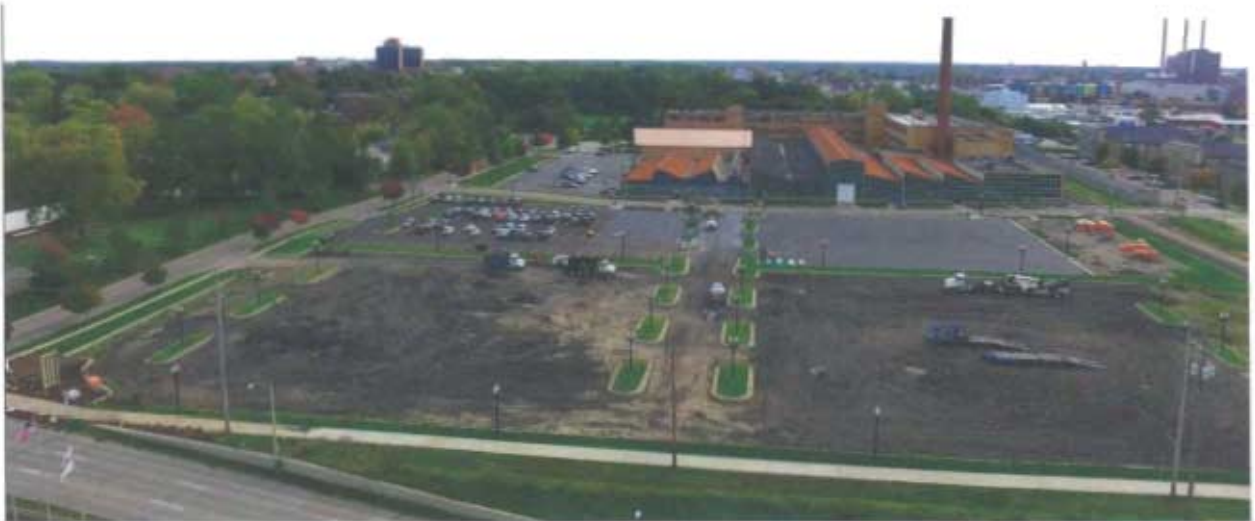
View from above Demmer looking South toward site.
