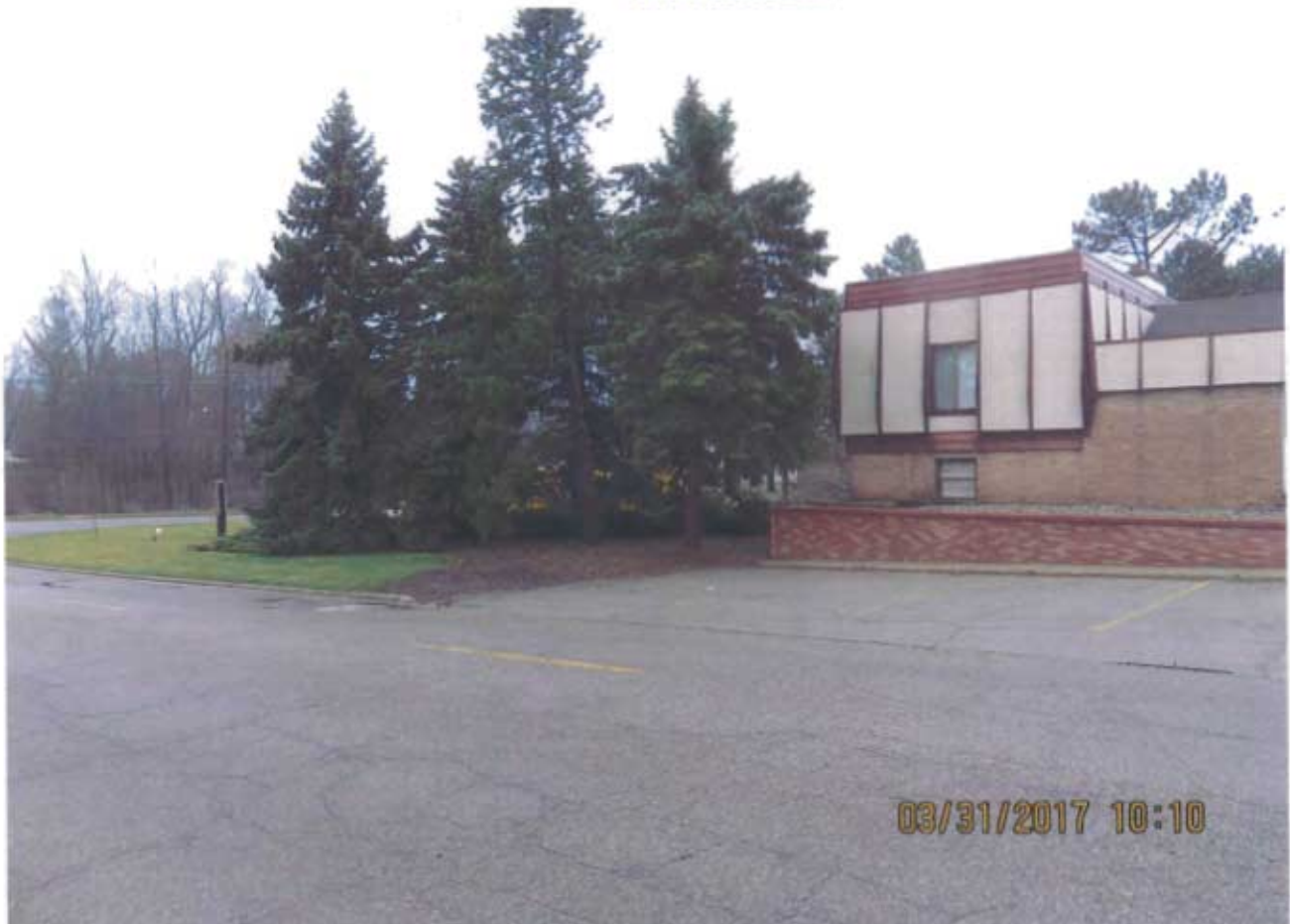
North Elevation (South end)
