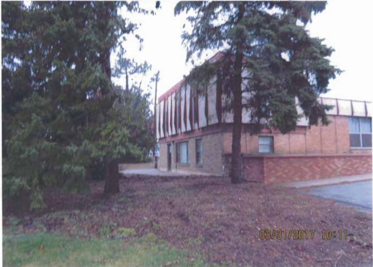
South East Corner
