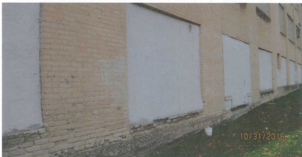
PHOTO: 2 DATE: 10/31/2016 SUBJECT: View of former windows filled-in with plaster.
