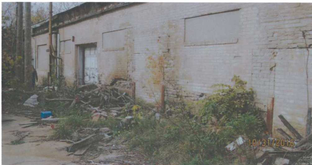
PHOTO: 6 DATE: 10/31/2016 SUBJECT: View of the south side of the building.
