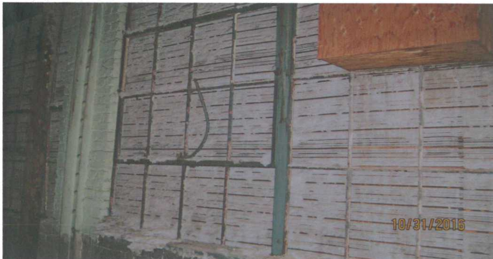
PHOTO: 8 DATE: 10/31/2016 SUBJECT: Interior view of former windows filled-in with plaster located on second floor.
