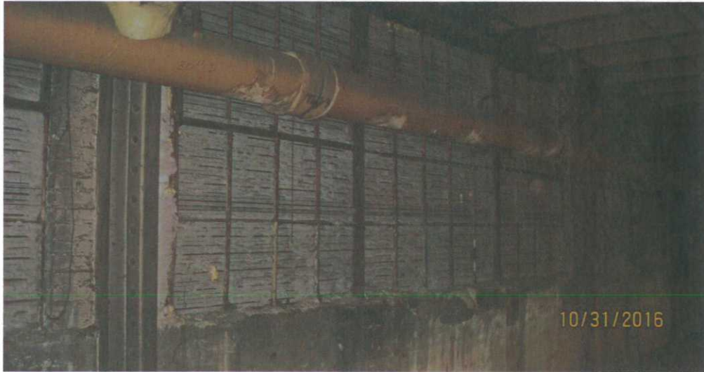
PHOTO: 9 DATE: 10/31/2016 SUBJECT: Interior view of former windows filled-in with plaster located on first floor.
