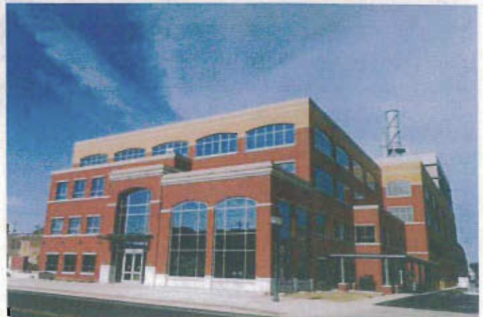
Near Board of Water & Light Power Station
