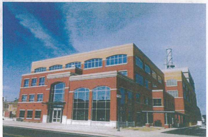
Near Board of Water & Light Power Station
