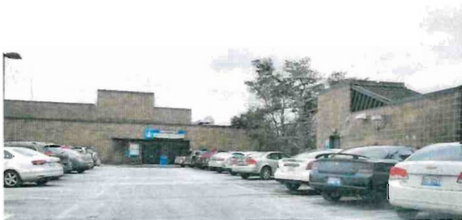
Photo 12: 3 rd Level Gannon Deck – looking south
