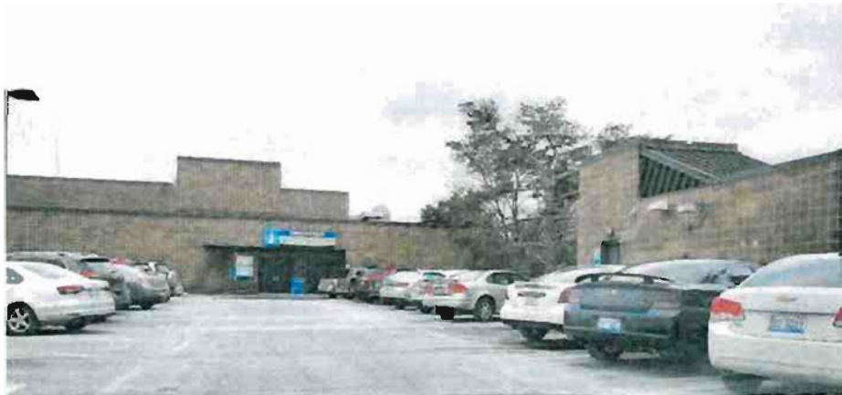
Photo 12: 3 rd Level Gannon Deck – looking south
