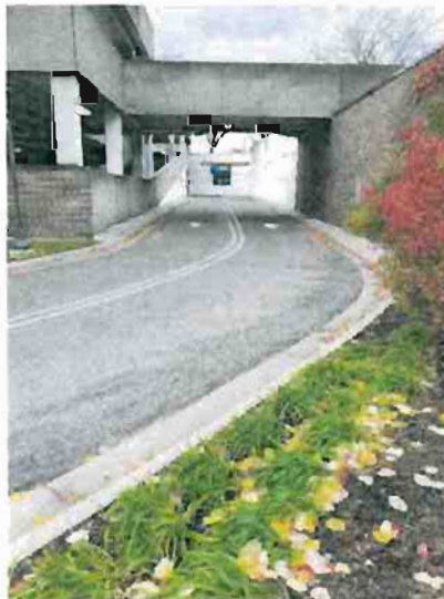
Photo 8: North Side Gannon Deck -- looking west along lower level entrance drive
