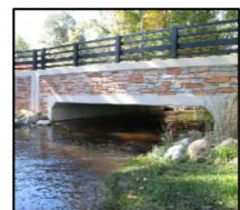
Figure 4: Three-sided box bridge
