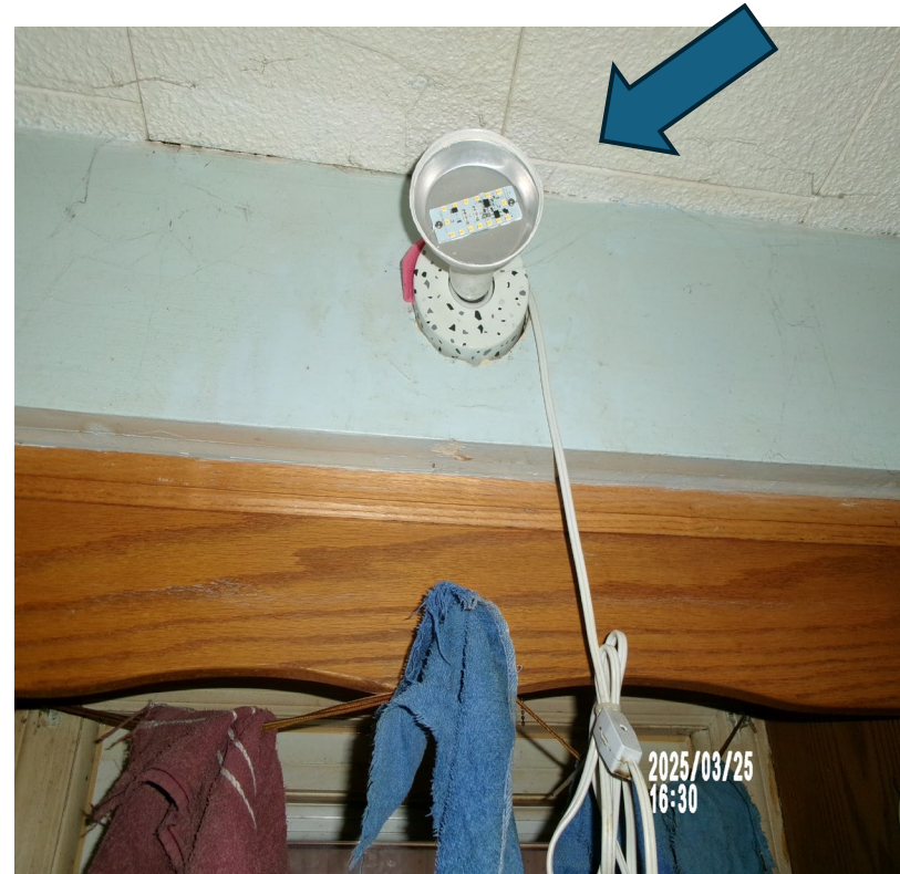
Flexible wire used to supply power to a light fixture in the kitchen area
