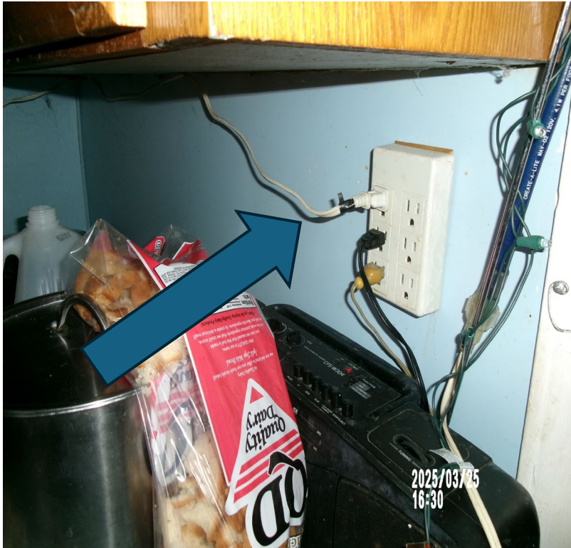
Flexible wire used to supply power to a light fixture in the kitchen area
