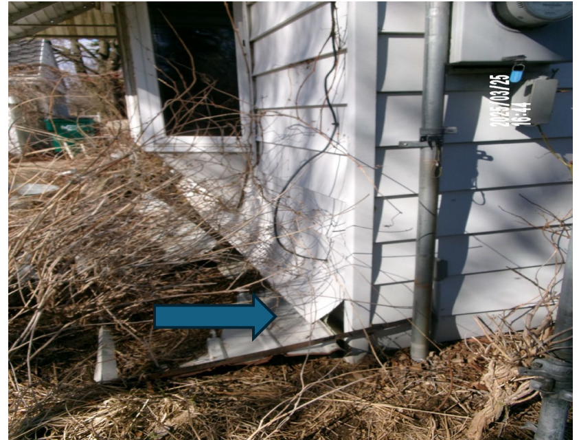
Rear of house signs of rear wall separation from structure
