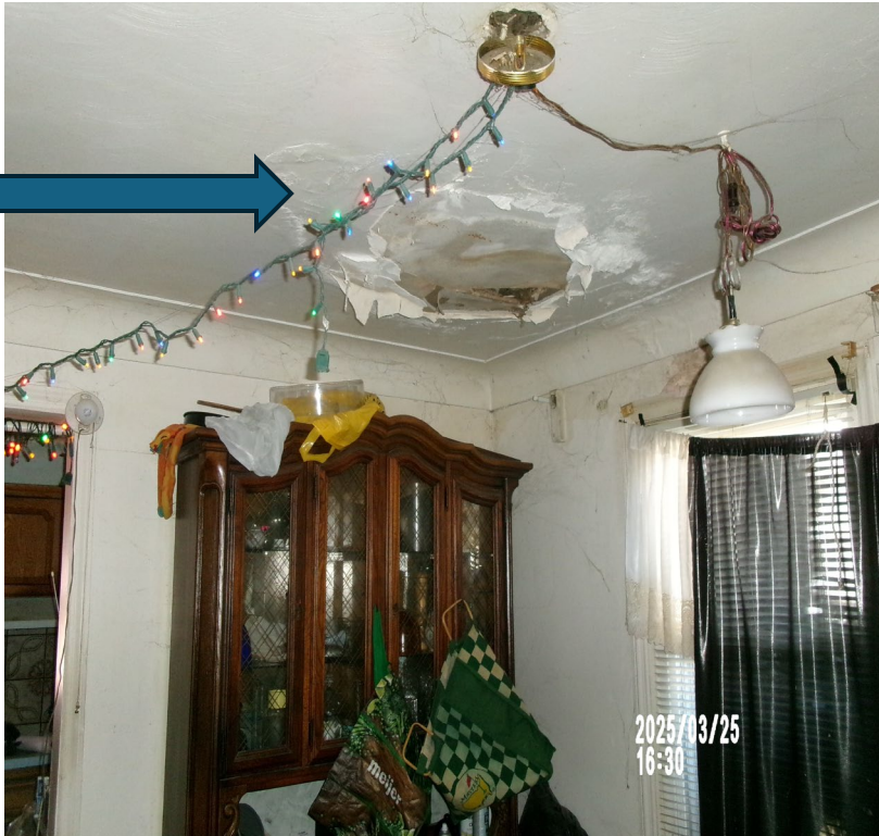
Water damage evidence from inside the structure at wall/ceiling area.
