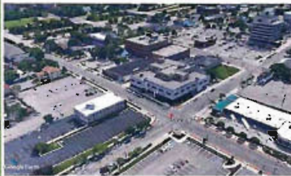
EXISTING SITE - ARIAL VIEW NW CORNER
