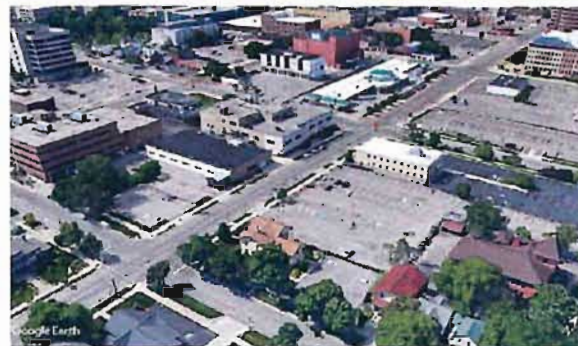
EXISTING SITE - ARIAL VIEW SW CORNER
