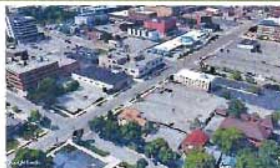
EXISTING SITE - ARIAL VIEW SW CORNER
