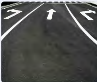
Dedicated Left and Right Turn at Intersections
