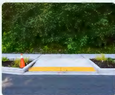
Curb Ramps/Sidewalk Utility Coordination
