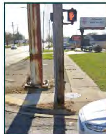
Figure 22 - Pedestrian signal at Pennsylvania Avenue
