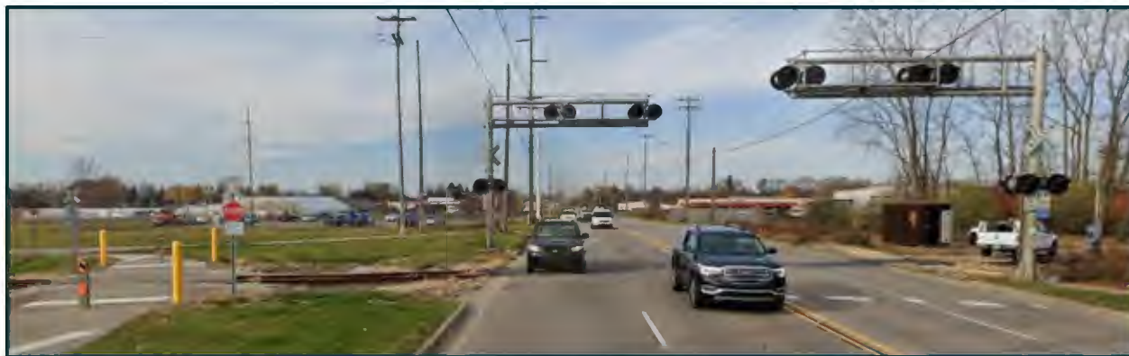
Figure 19 - Railroad crossing on Jolly Road, viewing west
