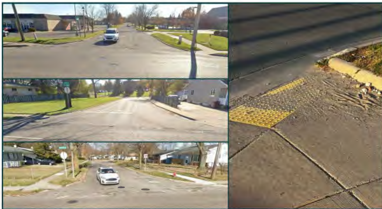
Figure 21 - Jolly Road crossing at Jolly Cedar Court (top), Battenfield Road (middle), and Southgate Avenue (bottom), covered detectable warning surface at Dunckel Road (right)
