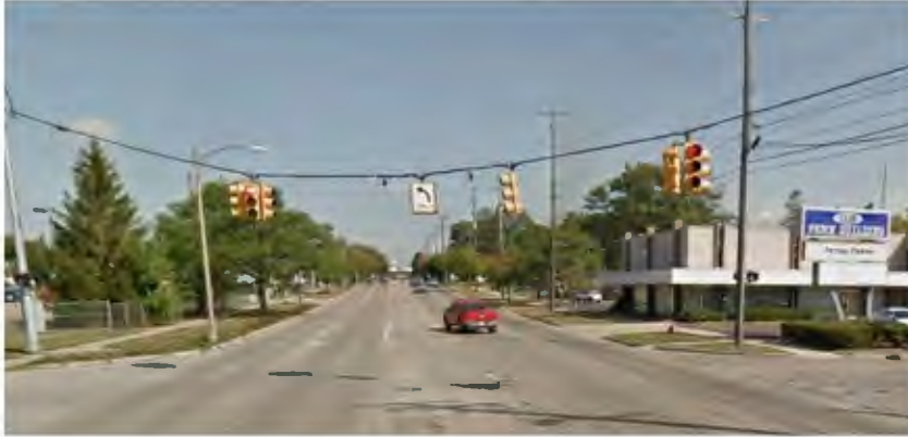
Figure 14: Diagonal Span Traffic Signal at Pennsylvania Avenue and Haco Street
