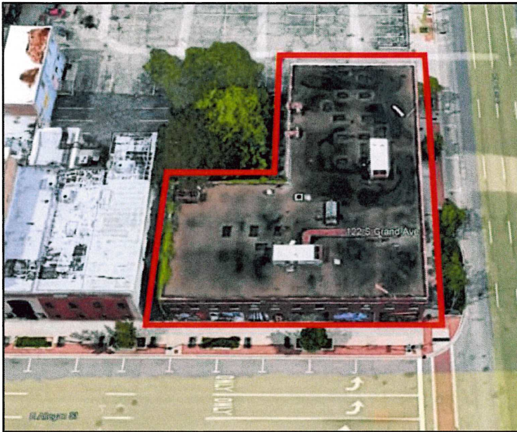
PHOTO NO. 1: Aerial view of Walter Neller building (within L-shaped red polygon).
