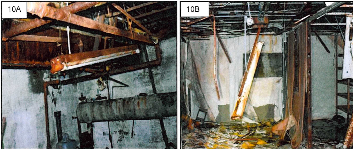
PHOTO NOS. 10A and 10B: Exposed portions of basement walls did not exhibit signs of structural inadequacy.
